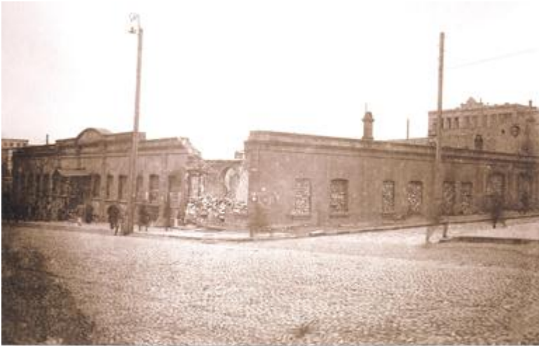
The view after the burning of the building of “Kaspi” newspaper in Nikolayev street
