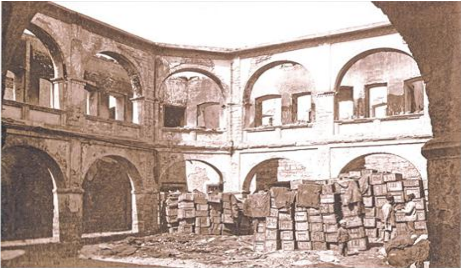
Bazarnaya street Khanlarov's house after the fire
